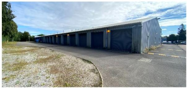
The subjects comprise a large single-storey motor dealership of steel portal frame construction with block infills, insulated composite cladding and glazed front elevation.
